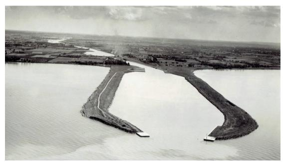
The Port Weller spits extend well out into Lake Ontario and were constructed between 1913 and 1932 (except for the war years when construction was paused) as part of the overall Fourth Welland Canal project. Rock and earth from the Canal excavation across the Niagara Peninsula was loaded onto rail cars which travelled the
